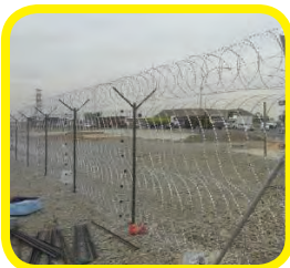
Razor Wire Fencing
